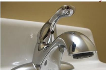
All of the plumbing fixtures in these buildings are low-flow. The faucets use 1.0 gallons of water per minute. The toilets have green, dual-flush handles. An upward flush uses 1.1 gallons of water and a downward flush uses 1.6 gallons. There are also low-flow shower heads. These fixtures are expected to reduce the building's potable water usage by about 40%.
