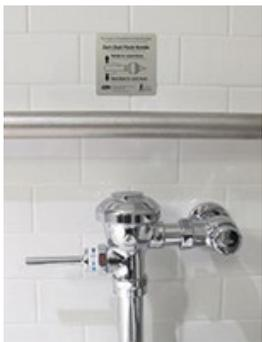
All of the plumbing fixtures in the building are low-flow. The lavatory faucets use 0.5 gallons of water per minute and sensors control how long they operate. The toilets have dual-flush handles, and the urinals use only 1 pint of water per flush. These fixtures are expected to reduce the building's potable water usage by about 36%.
