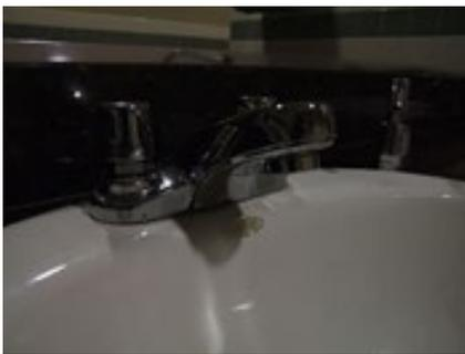
The plumbing fixtures in Lakeside Dining Hall are low-flow. The lavatory faucets use 0.5 gallons of water per minute and sensors control how long they operate. The toilets are dual-flush, and the urinals use only 1 pint of water per flush. The low-flow plumbing fixtures are expected to reduce the building's potable water usage by 33% or over 190,000 gallons/year.
