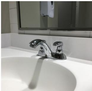
The restroom plumbing fixtures in the building are low-flow. The lavatory faucets use less than 1 gallon of water per minute, toilets have dual-flush handles and the urinals use only 1 pint of water per flush. These fixtures are expected to reduce the building's potable water usage by about 32%. The landscaping around the building is designed to minimize the need for irrigation.
