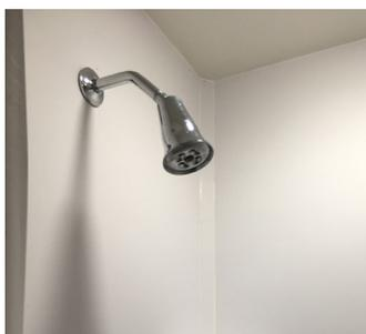
The buildings have low-flow plumbing fixtures throughout. The lavatory faucets use 0.5 gallons of water per minute, and the shower heads are 1.6 gallons of water per minute. The toilets have dual-flush handles, and the urinals use only 1 pint of water per flush. These fixtures are expected to reduce the buildings' overall potable water usage by more than 40%.
